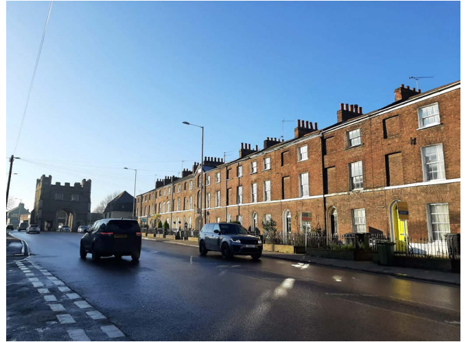
Grade II Listed Buckingham Terrace, London Road
